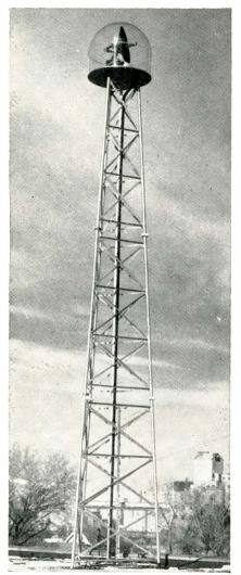
This radar weather tower of KSTP-TV. Minneapolis, uses the 3 lower sections of the ROHN "Self-Supporting" tower. Note construction, design and size.)
