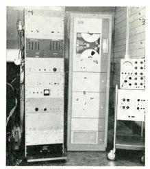
Surface ignition detection instrumentation, including peak pressure pulse generator and data read-out rack, two channel magnetic tape recorder, and calibrating oscilloscope.
