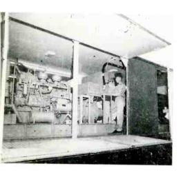
(Left) Sideflaps peeled back, power truck is ready SUDDIV power to Frescanar under field conditions.
