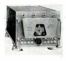
channels, the receiver provides coverage of the 1000 to 12,000 MC spectrum. Total frequency coverage is divided in three 2:1 bands and one 1.5:1 band. Each channel provides a stretched (300  $\mu$ sec) output for recording and aural monitoring, and an unstretched output for pulse width and prf analysis. Granger Assoc., 966 Commercial St., Palo Alto, Calif.
