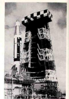
Gantry tower used in readying the Atlas ICBM is rolled away from launch stand, leaving missile poised for flight, at the AFMTC, Cape Canaveral, Fla. Convair-Astronautics designed and built the Atlas.
