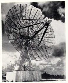
Higher than a 7-story building this giant 60-ft wide antenna built for ARDC by Radiation Inc. at Melbourne, Fla., is one of five that will pick up telemetering information from highflying-ballistic missiles.
