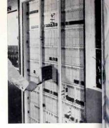
Fig. 10: Printed circuits, transistors, pl in boards are combined to form the Digit automatic machine controls.
