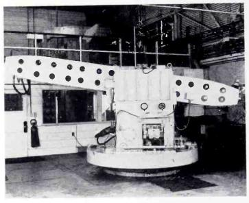
(Above) Hydrodynamic Simulator at Naval Ordnance Test Station, Pasadena, Calif., tests torpedoes under simulated sea environment.
