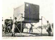
An easily assembled lifting device simplifies the Army's task of raising this Craig Helicop-Hut to level of truck bed. Shelters are designed to house complete radar, microwave or other installations
