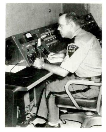
(Right) Two separate duplex VHF systems serve the Indiana State Police and turn pike maintenance personnel. The two transmitters are connected to one antenna, through tuned cavities. The receivers are similarly cavity-linked to one antenna. Interaction is negligible.
