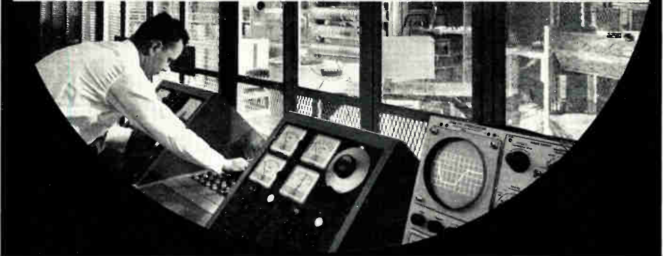
Howard Jessup, Westinghouse Design Engineer, testing relatively high power interstage pulse transformers on the new line-type pulse modulator designed by Mansom Laboratories Incorporated, Stamford, Connecticut.
