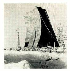
White Alice, Alaska's new tropospheric scatter communications system, uses 60-foot antennas such as this. White Alice is a project of Radio Engineering Laboratories.
