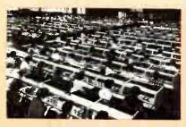
"area cleaning"—new installation of complete air conditioning and air filtering keeps areas, such as mounting department, relatively free from dirt and dust.
