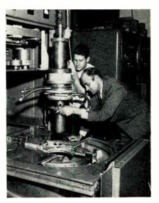
Signal Corps engineer Ralph Johnson inspects fittings as William Mitchel, of Continental Electronics, Inc. lowers a 150-pound tube into its socket in Pentagon's new transmitter
