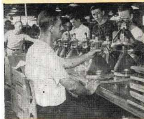
TV components that are sub-assemblies are constructed on auxiliary production lines. Riveting tube sockets and terminal strips onto the main chassis is primary operation
