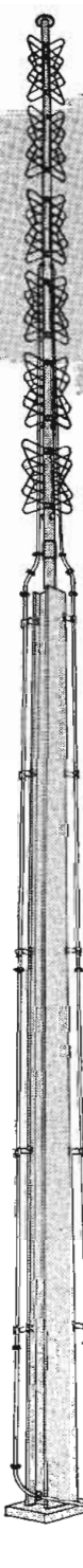
Television antenna of WGN-TV — Chicago's newest and most powerful television station—showing Andrew 1-5/8" flanged television transmission line.
