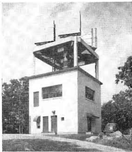
One of the seven hilltop relay stations in the 220-mile stretch between New York and Boston on the Bell System TV relay
