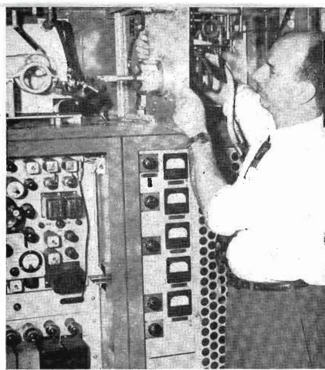
WNBW depends upon an RCA type 8D21 tube in which all elements are internally water-cooled. Transmitter is on Channel 4
