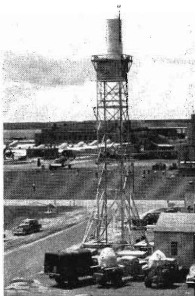
Fig. 10—The height-finder tower, separated by 500 ft. from the indicator room in the airport control tower
