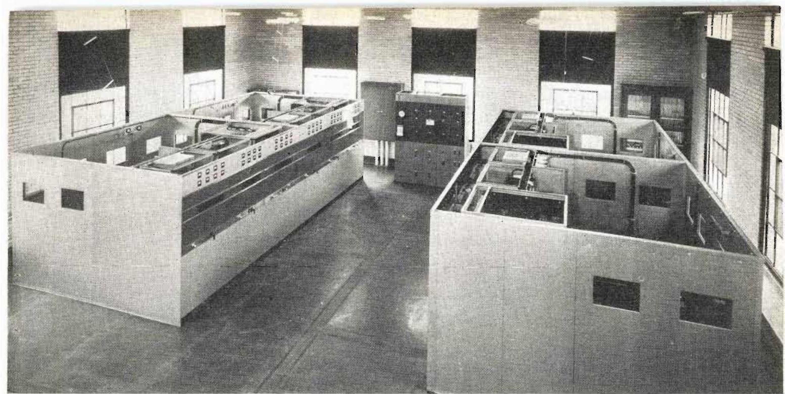
Interior view of the National Bureau of Standards radio station showing 4 of the 8 transmitters. In addition to standard frequency signals and time and musical pitch, warnings of ionosphere and propagation disturbances are broadcast
