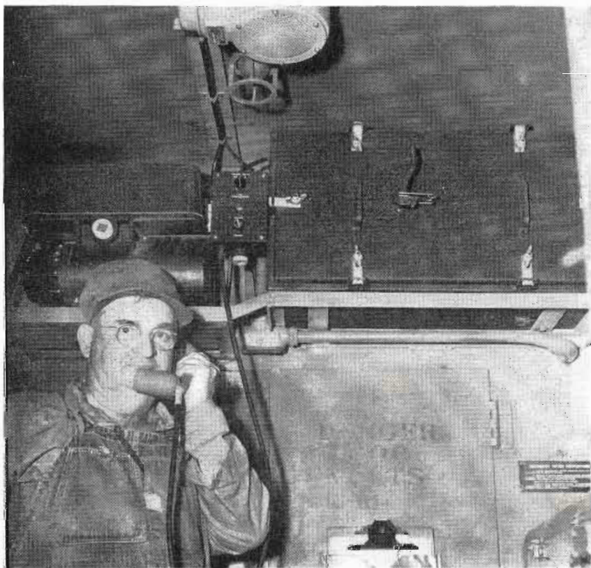
Typical installation of Bendix VHF two-way communications equipment on one of the Frisco Diesel switching engines at Springfield
