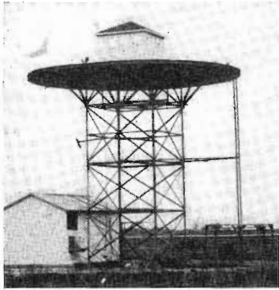
Omni-range antenna housing, screen
