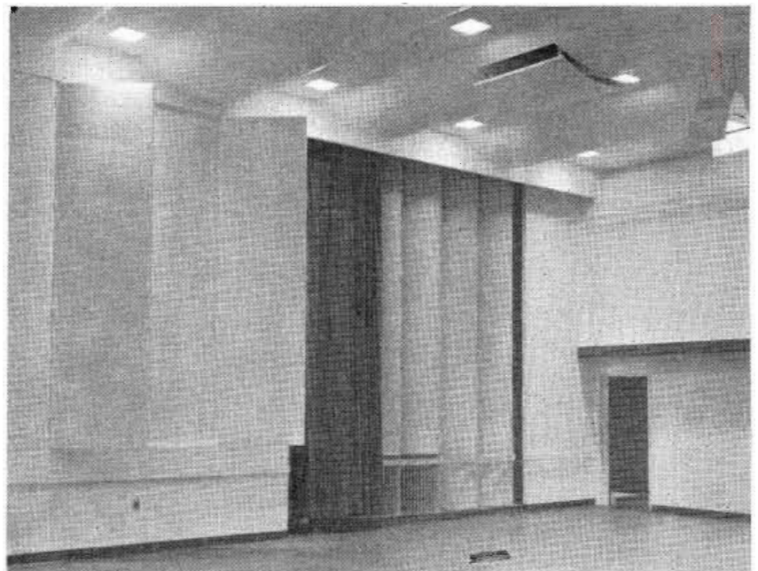
Fig. 3—Note heavy draperies and hinged “acoustical” panels for response changes
