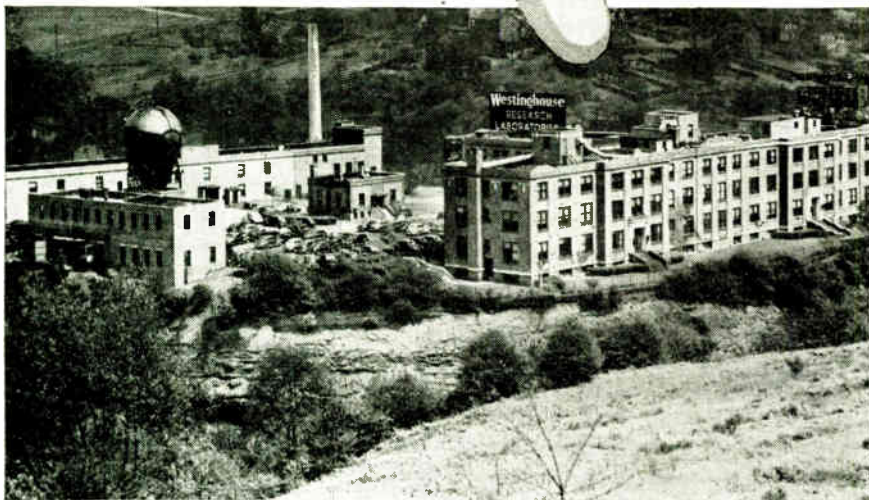
Part of Westinghouse research laboratories at East Pittsburgh, Pa.
