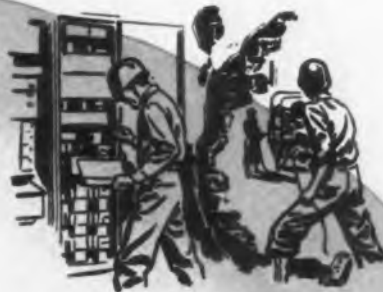
Bell Laboratories and Western Electric furnished revolutionary carrier telephone terminal equipment in great quantities—all "packaged" for quick installation in the field.
