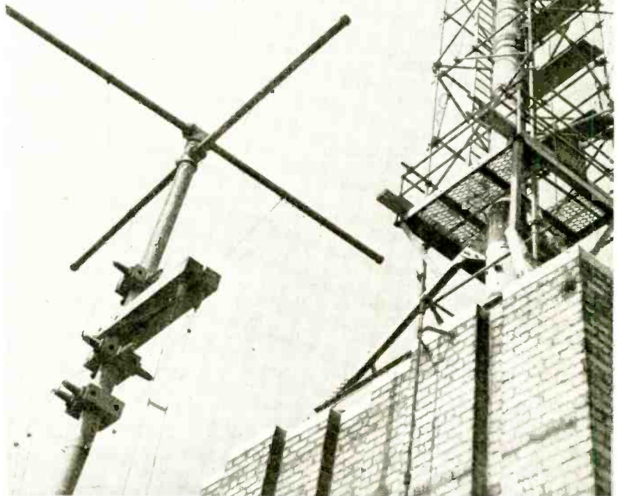
Fig. 3—The old antenna, erected just before the war and used since, was a simple, single bay radiator
