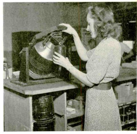
10 Idea for handling inflammable or corrosive solvents eliminates manual lifting, promotes safety, and speeds entire process of filling girls' individual containers at a Westinghouse plant. The safety can-tilting stand incorporates lever to pull stopper automatically
