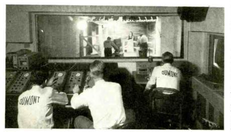
Newly completed studio and control room facilities at WABD, the Du Mont tele station in New York City. Lamp banks are incandescent and adjustable. Two dolly-type cameras are used
