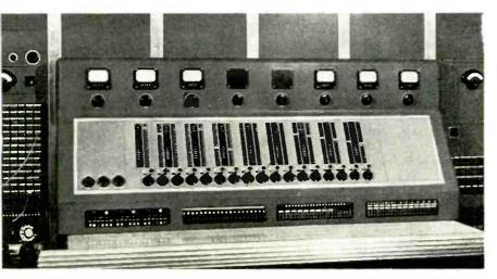
In the KHJ master control room there are 17 separate switching systems which can be individually controlled or as many as desired group switched by a master button. The board is used to route programs north, south and east to the Don Lee network, and east to Mutual
