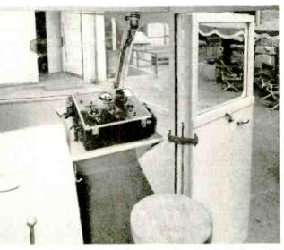
Recording operator's position from the inside in a wide compartment which he shares with the vehicle's driver
