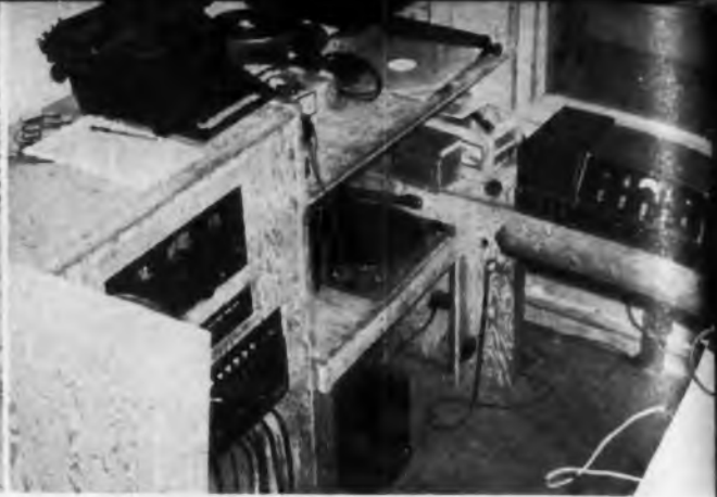
A corner of the master control room in the North African station. Engineers had to rely mostly on plywood for construction
