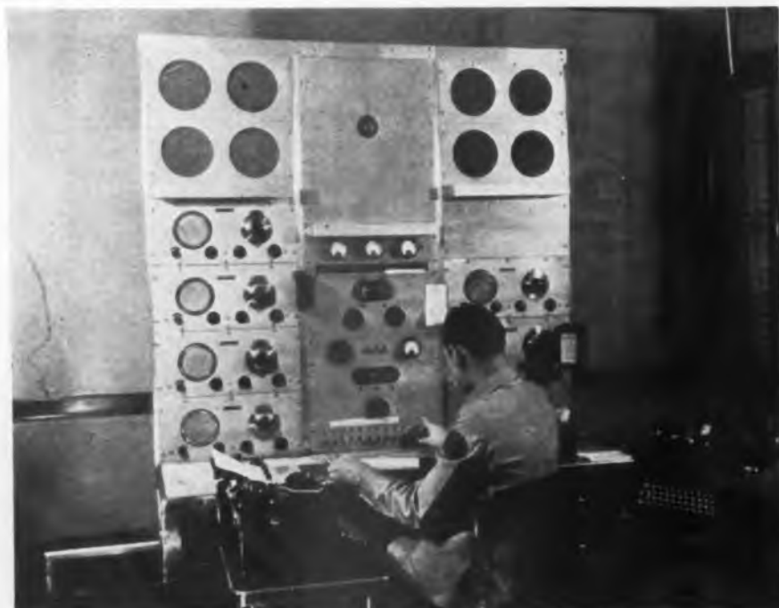
Below is a view of part of the radiophone control panel at State headquarters in Lansing. At right is shown one of four remote controlled unattended 250-watt transmitters used to cover the city of Detroit
