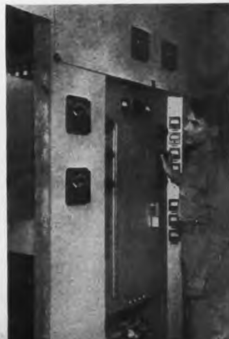
Front view of high frequency channel of Westinghouse 50GH
