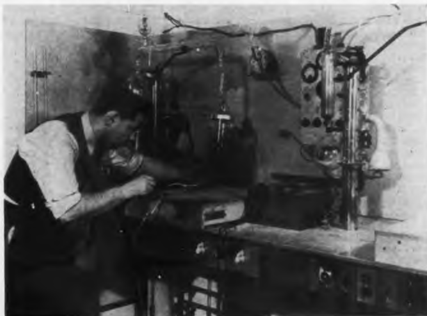
Early stage in manufacture of television dissector tubes at Farnsworth. Installation of Precipitron solved cathode dust spotting problem
