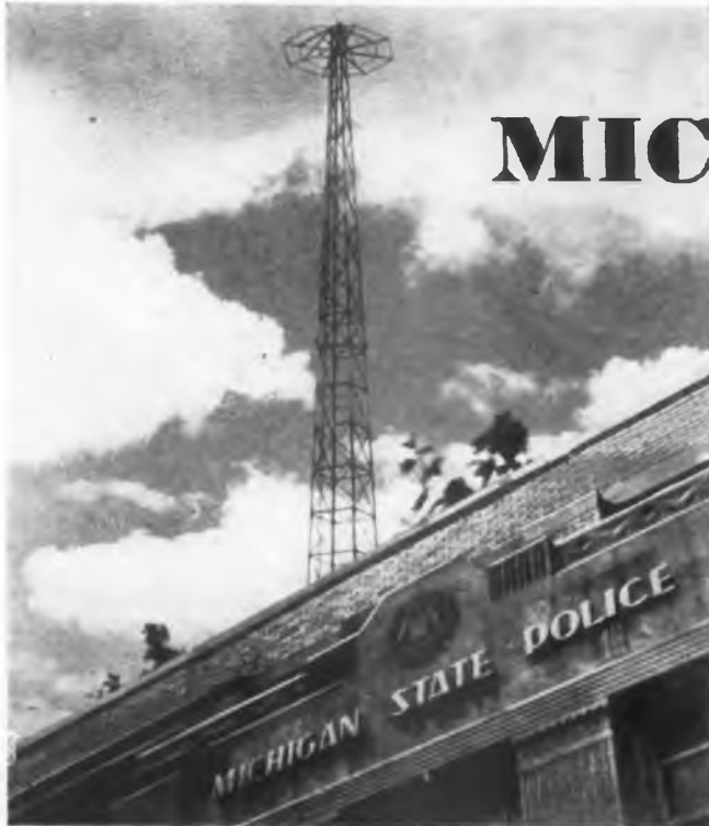
Administration bldg., headquarters of Michigan's police net
