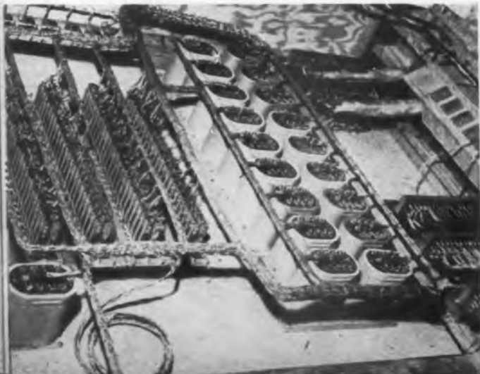
Back of the panels in the master control room of the North Africa United Nations station reveals more plywood construction, this time holding the wiring (left) and the line amplifiers
