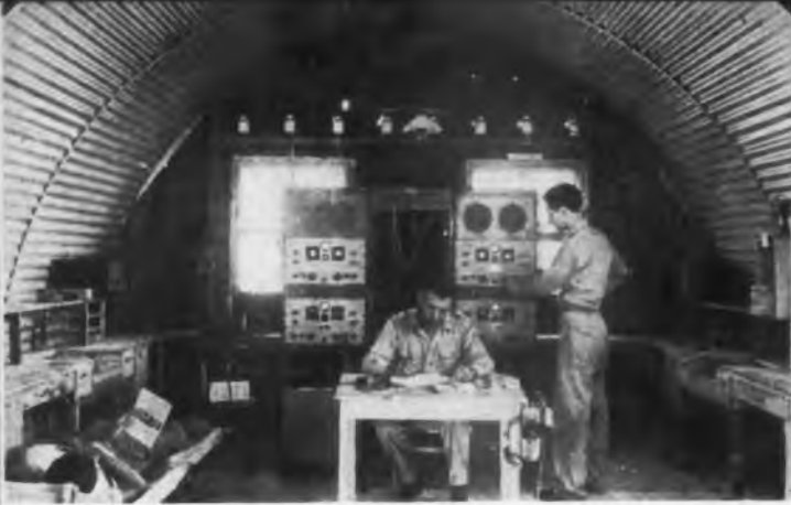
One end of Nissen hut installation showing dual-diversity receivers used for relaying programs originating in New York
