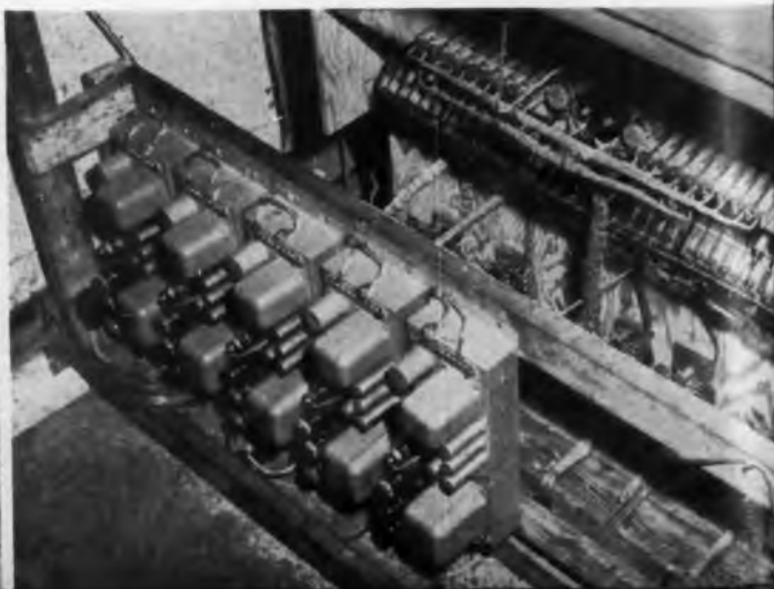
Back of the panels in the master control room of the North Africa United Nations station reveals more plywood construction, this time holding the wiring (left) and the line amplifiers
