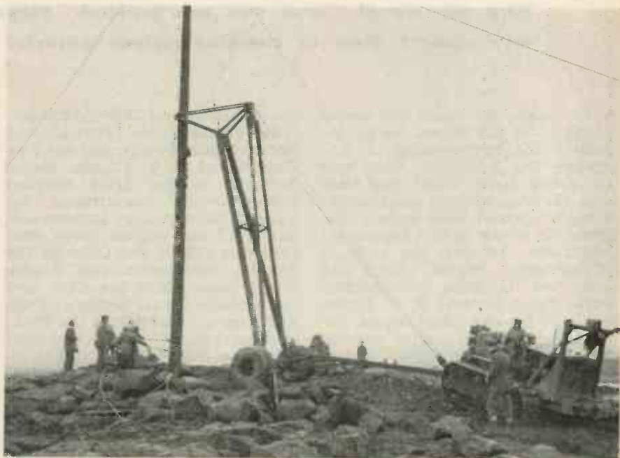
Anchoring antennas in rock was only one of the many problems involved in construction of the Signal Corps' six new long wave transmitters in the Arctic
