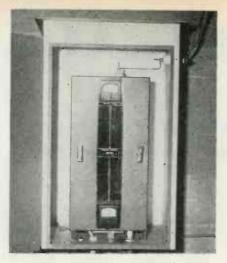
ANTENNA tuner is located indoors at the base of the tower
