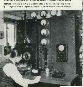
MEASURING characteristics of a special instrument in the completely isolated high-frequency cage
