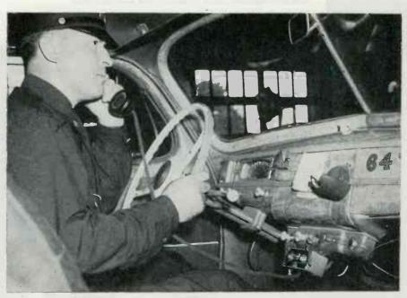
EACH of the 70 mobile police units carries AM receiving equipment and for talk-back operators rely on 25-watt FM transmitters on 35.1 megacycles
