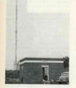
RECEIVING antenna is mounted on 200 ft. pole above another antenna
