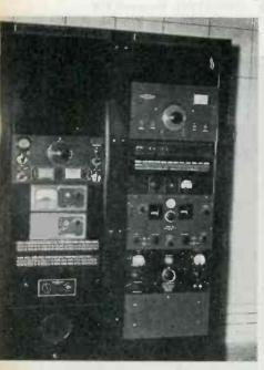
AMPLIFIER and patch panels containing terminations for all receiver lines
