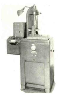
INVOLUTE MEASURING machine equipped with GE chart type electronic recording device manufactured by Fellows Gear Shaper Co.
