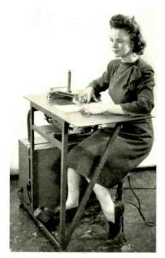
RADIO-FREQUENCY current stitches a thin solid seam that is both air- and water-tight. Developed by RCA for the plastics industry in fabricating thermoplastic materials
