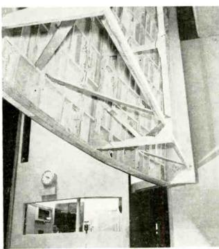
CONSTRUCTION DETAILS are seen above of the heavy drop. Below, the elevation sketch of the stage shows how the exponential-horn form has also been applied to the vertical section of the new WOR theater studio.
