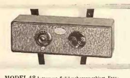
MODEL 48 battery set. Solid inabogany cabinet. FUL-VISION Dial. Two stages of T. R. F. In conjunction with Atwater Kent coupling circuit, detector and two stages of A. F. Six tubes required. Without tubes or hatteries, \$49
