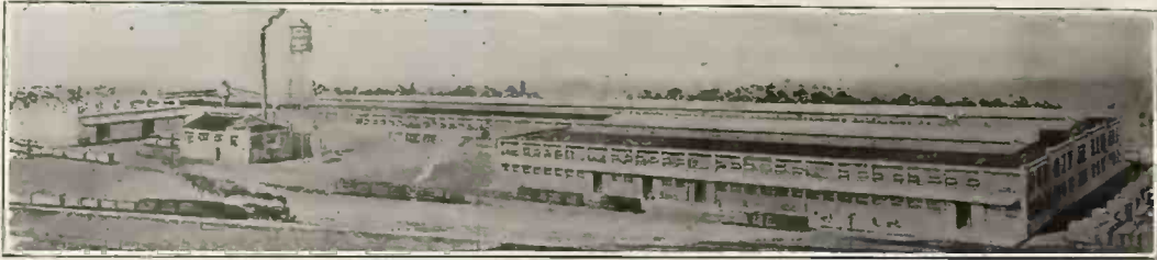
One of the Showers Bros. Co.'s Large Cabinet-Making Plants
