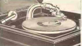
Showing Reproducer of Jewel Needle Equipment in Position for Playing Edison Record With Fibre Needle.
