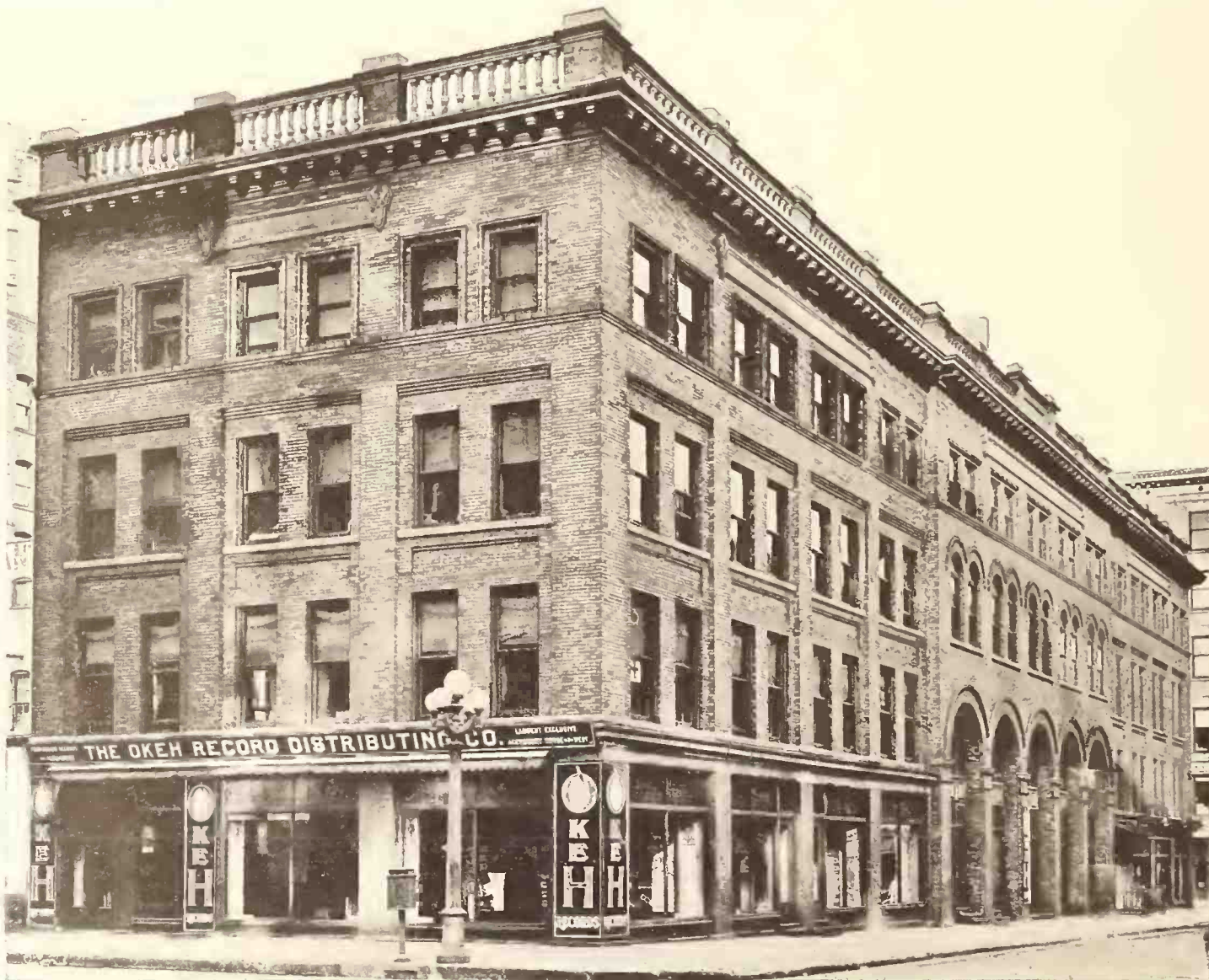
OKEH BUILDING, GRAND RAPIDS
