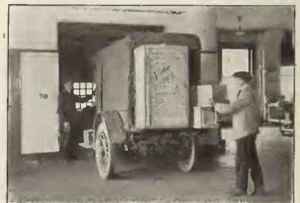
Loading Truck Right on Stock Floor
