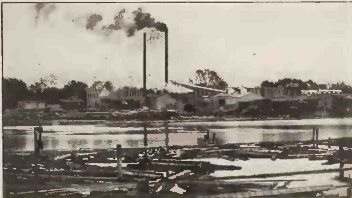
View of the Veneer Mill
