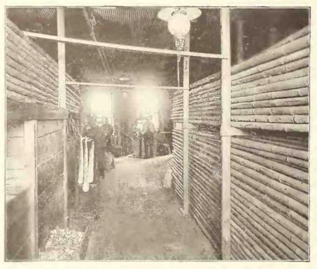
5,000 poles—20 feet long and 3 inches in diameter—are here stacked until thoroughly dried, then sawed between joints.
