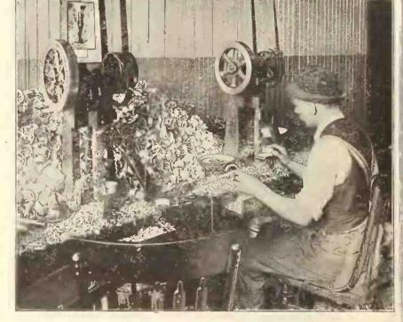
Blocks, sawed from joints, are here shown being fed into specially devised splitting machines. Capacity of each machine—162 needles per minute.
