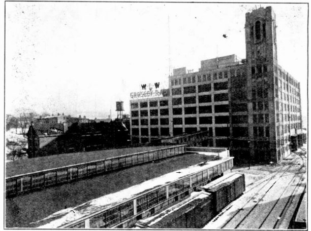
New Crosley Addition Rapidly Nearing Completion
