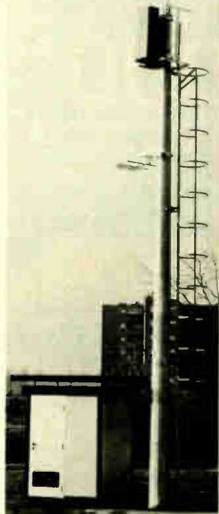
Fully pre-assembled box and standard pole for telecommunication systems
