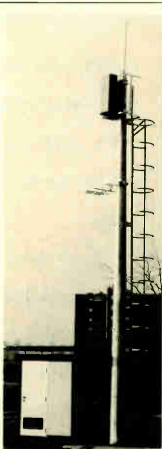
Fully pre-assembled box and standard pole for telecommunication systems
