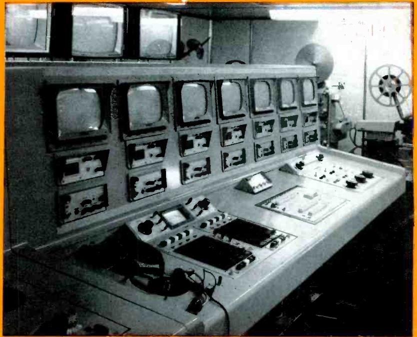
Control panel on liner "France"
