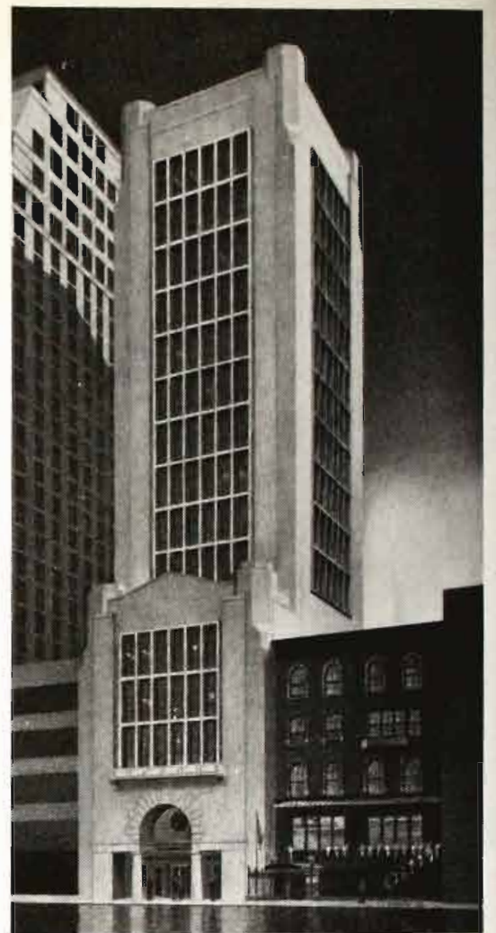
The new home for the Museum of Broadcasting.
