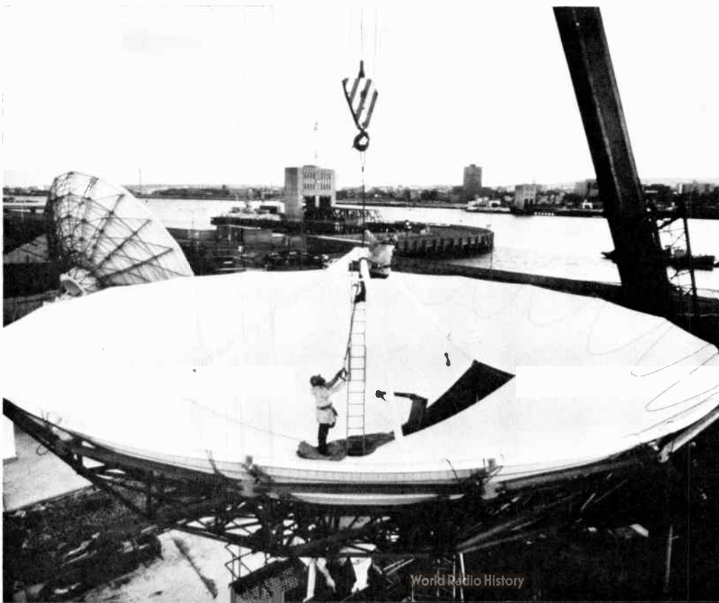
Aerial 2, the second of six huge dishes being installed at London Teleport, North Woolwich. It is expected to provide London's business community with a full range of advanced communications services.
