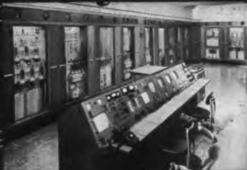
Transmitter room of WOR-TV's new Empire State 50 KW transmitter. 130 KW ERP. 100% air cooled. Completely self-contained. Equipment throughout by Standard Electronics.
