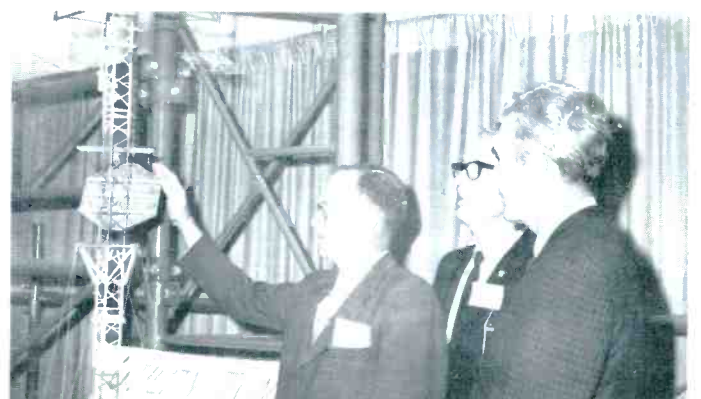
UTILITY TOWER: David P. Callahan, Rowley United Theatres; D. E. Neilson and Bud Duvall of Utility.
