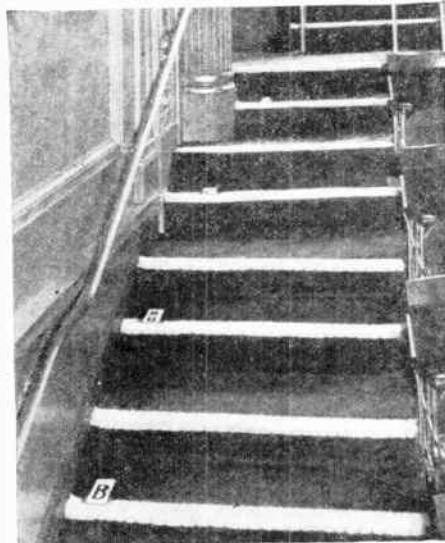
In a theatre Osglim lamps indicate the seats by illuminating letters on glass, behind which the lamps are placed. It will be observed that there is one letter for each second step, as there are two steps for one row of seats.
