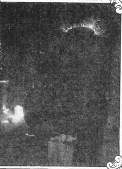
A sustained arc at about 970,000 volts across a gap of 109 in. The cobweb effect noticeable in the discharge is caused by the low frequency alternations of the current. Each white line indicates the crest of a current wave.
