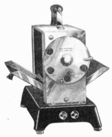
This self-timing electric toaster will be halled by all housewives as a boon to domestle felicity. When the proper degree of toasting is reached an adjustable timing mechanism drops the wings upon which the slices of bread are carried.
