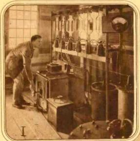
Left: The 30 K.W. 15,000 volt three phase rectifier for 107 meter wave-length. At the General Electric Company's Schenectady Plant.
