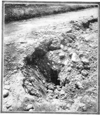
An unprecedented display of the destructive power of a lightning stroke is illustrated above. A 20-inch cast iron gas main had been installed but fortunately was not in service. The lightning struck, tore the pipe to pieces, opened a great cavity in the earth, and had the pipe been in use for conveying gas it is hard to say what the result would have been. The pipe was three feet underground.
