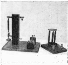
A very delicate microphone can be constructed with a double pointed carbon rod supported between two carbon discs,
