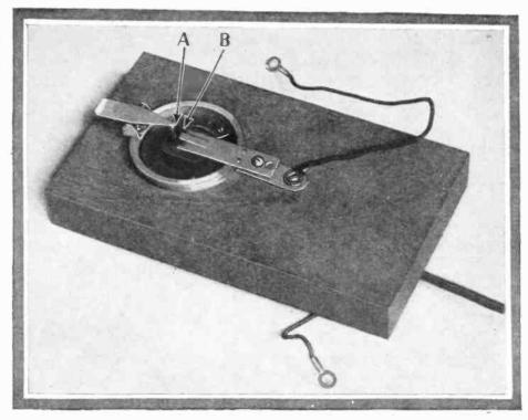
A microphone amplifier that operates on the Taulelgne principle. A microphone contact is obtained between the two carbon electrodes A and B. The lower one is actuated by the telephone.
