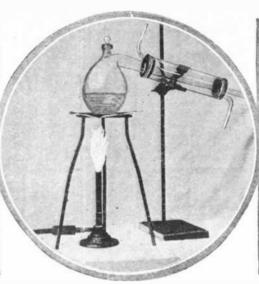
Making nitric acid from sodium mitrate, the so-called Chile saltpetre. Note the simple condenser.
