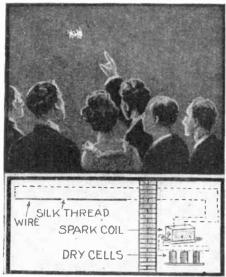
Mysterious "wireless" sparks are produced before the eyes of wondering spectators who do not suspect that wires, rendered invisible in the orange illumination, are stretched across the room and connected to a remote spark coil.
