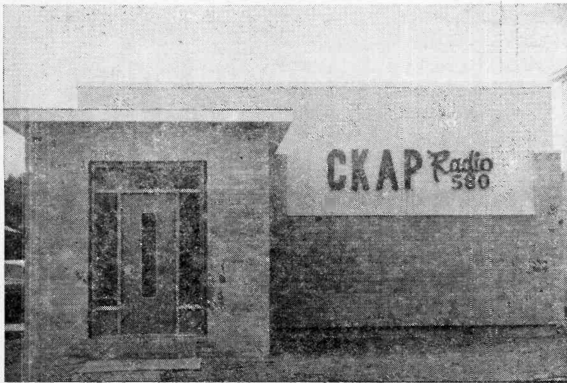
Radio 580, CKAP, Kapuskasing, boasts the most modern studio facilities in Northern Ontario. Located at 24 Byng Avenue, this fine building houses dual control rooms, an announce studio, a newsroom, and general administrative offices. Beginning Monday, August 2nd, office hours will be from 9:00 a.m. to 5:00 p.m. daily. 'Open House' will begin July 31st, and will extend throughout the entire month of August.
