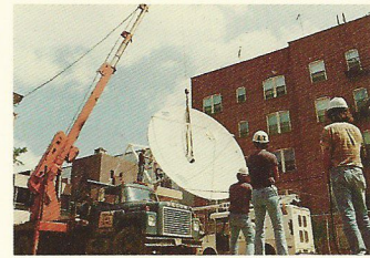
A dish antenna goes into place during the construction of the company's Suburban Cablevision cable-TV system in New Jersey in the middle 1970s.
