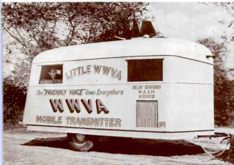
This is "Little WWVA", a mobile unit carrying 2 short wave transmitters that enabled WWVA to broadcast from remote locations. It went into service in October 1937. Engineers Glenn Boundy, in window, Jack Supler, top, and Bill McGlumphy (not pictured) traveled with the unit as it toured the WWVA listening area.
