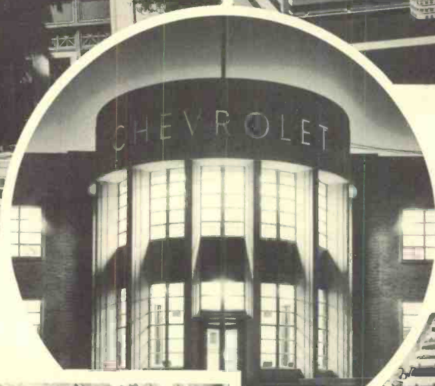
Strikingly handsome is this night view, the main entrance of the new Chevrolet Assembly plant.
