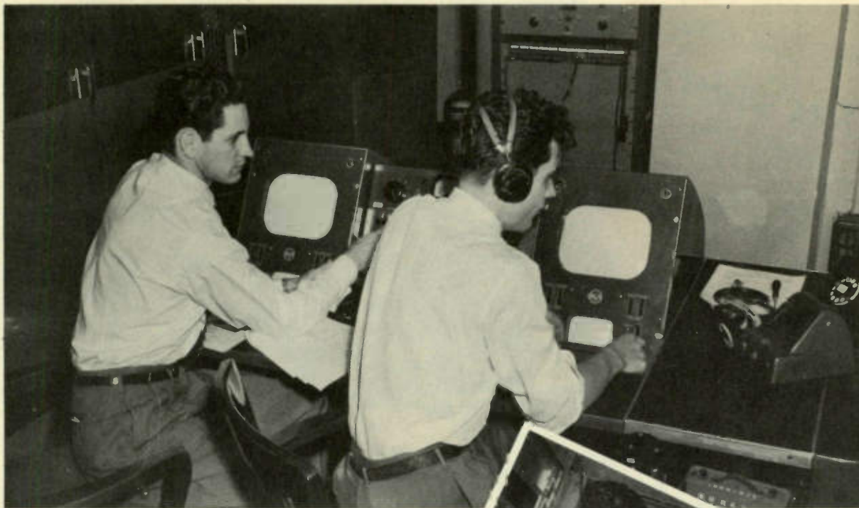
Seated at the WTVN control-console are Engineers Cal Garrison and Dale Lardie. Both are busy shading WTVN's picture pattern while checking the film monitor on the left and the master monitor on the right.
