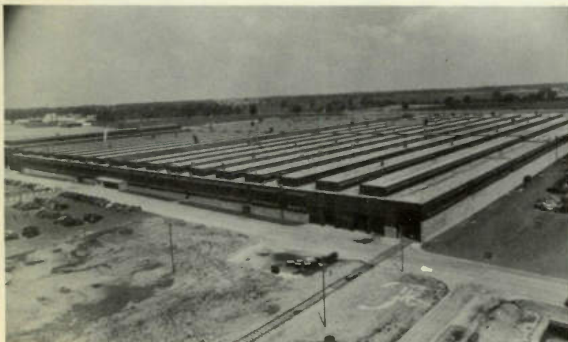
The Temstedt Mfg. Division of the General Motors Corporation, makes the body hardware for all G.M. cars. Under its roof are 16 acres of space.
