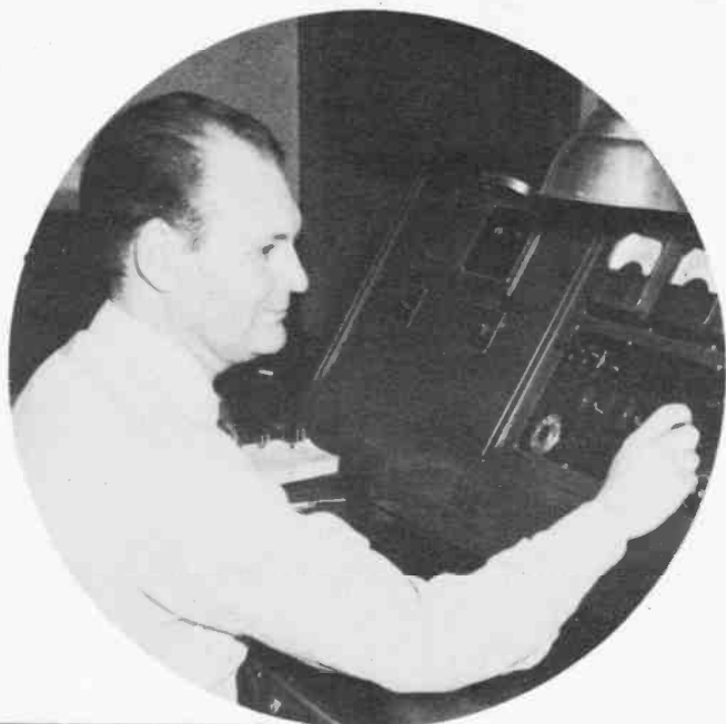
Vernon Goforth, Transmitter Supervisor, keeps constant watch on transmitter panel board to insure WSPA listeners the finest reception.
