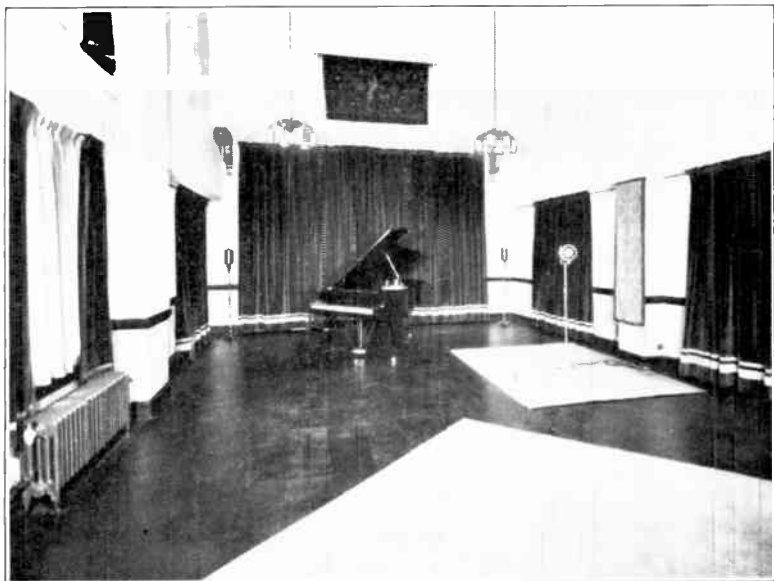
The GREEN ROOM, the largest studio at WRC. The blended gold and green tints of the walls and ceiling, the rich green velour drapes, make this a truly beautiful room. Four amber leaded glass casement windows, which diffuse a soft, warm light, are also hung in green velour. Two interesting brocades on the wall add a touch of true beauty.
