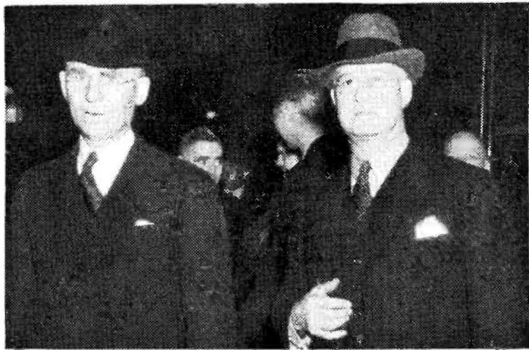
At noon, on February 22, Governor Roy L. Cochran of Nebraska turned the throttle control which efficiently started the new one-million-six-hundred-thousand-dollar service addition to the Nebraska Power Company plant in Omaha. As he turned the throttle, James E. Davidson (at right), president of the Nebraska Power Company, proudly watched 40,000 more horsepower added to the capacity of the power company's present plant. This ceremony was broadcast over WOW, and was handled by Foster May.
