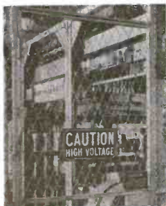
A safety gate back of the transmitter. If this gate is opened while transmitter is in operation, all current is automatically shut off.
