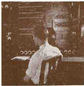
This is the central control room at the WLW studios. Through this control-board all programs are regulated and cleared to the WLW transmitter located at Mason, Ohio.
