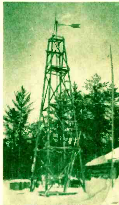
Ryburn's home made power plant.
