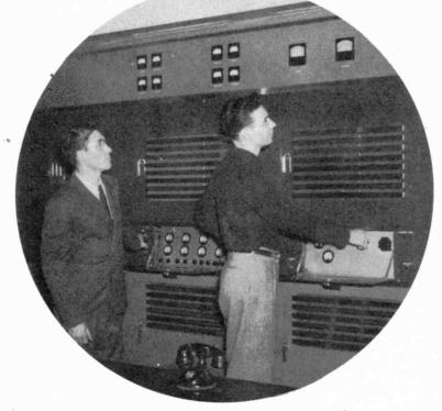
The huge RCA transmitter panel covers the entire wall of the building. About half of it is shown here as some of the readings are noted on the intricate dial system by Engineers KENNETH MOORE (left) and ARTHUR COVELL. It's a tiring, meticulous and often thankless job, being an Engineer but without them, the efforts of the entire remaining staff would be wasted.
